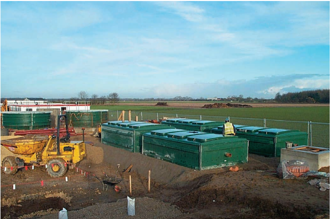
Bishop Dyke 2 (courtesy MWH).
