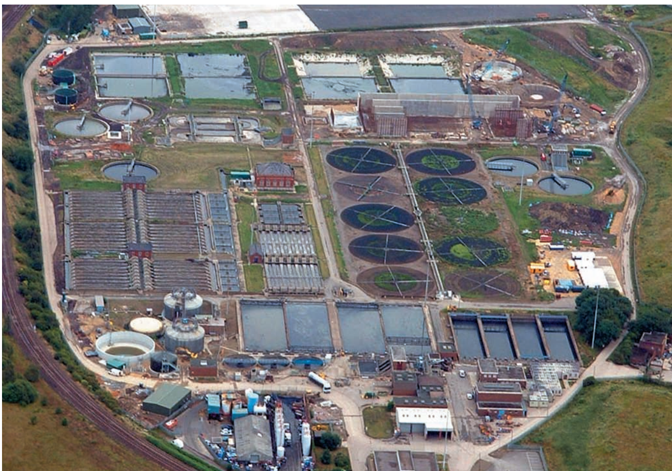
Calder Vale STW - aerial view of upgrades under construction (courtesy John Gruson BEng, BSc).
