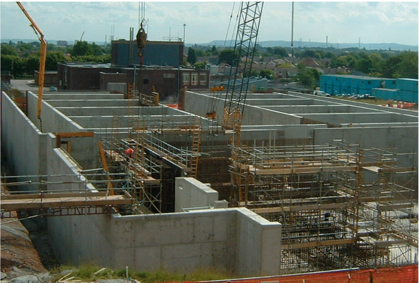
Upgrade work ongoing at Sutton Hall WTW.(courtesy Degremont)
