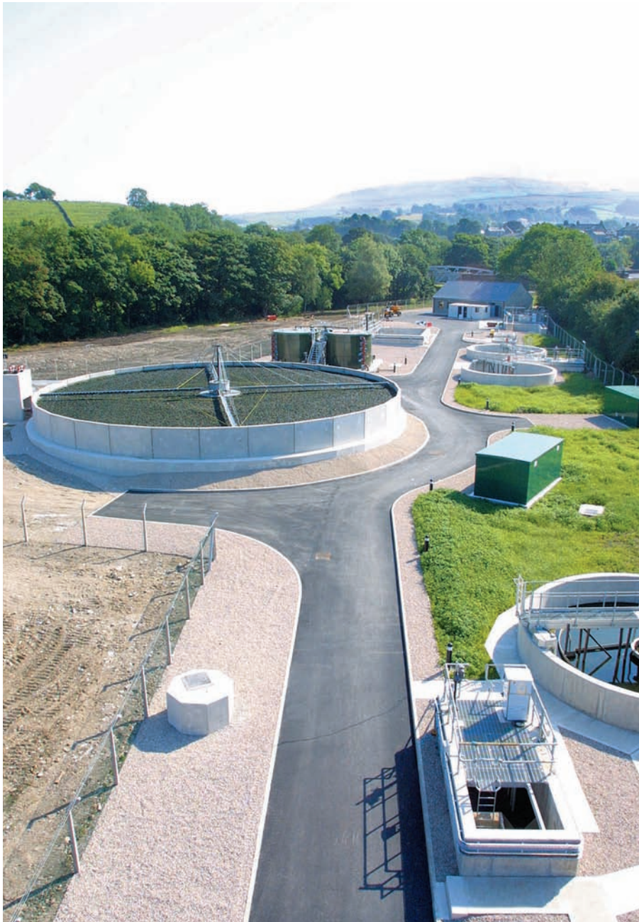
Ingleton WwTW (courtesy KMI Water & United Utilities).
