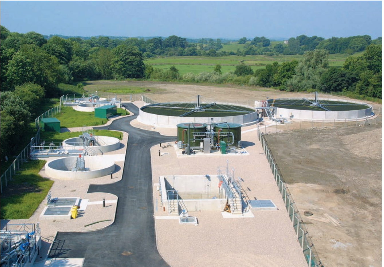
Ingleton WwTW (courtesy KMI Water & United Utilities).
