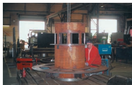
Part of the new internal structure
