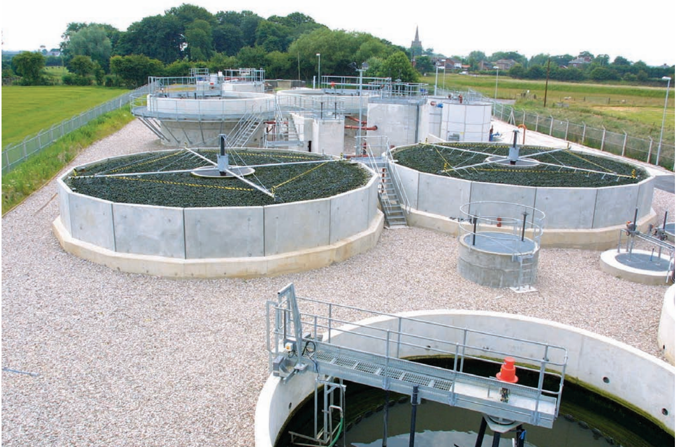
Pilling WwTW (courtesy KMI Water & United Utilities).
