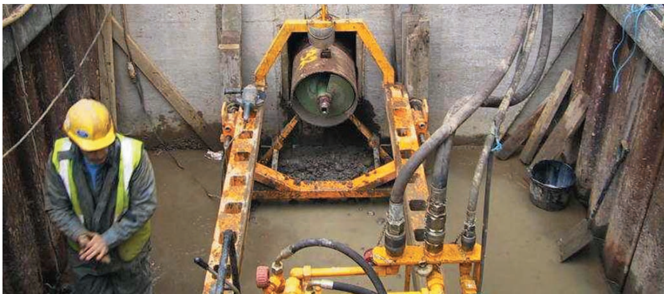
Cockshot Farm – directional drilling (courtesy Southern Water)
