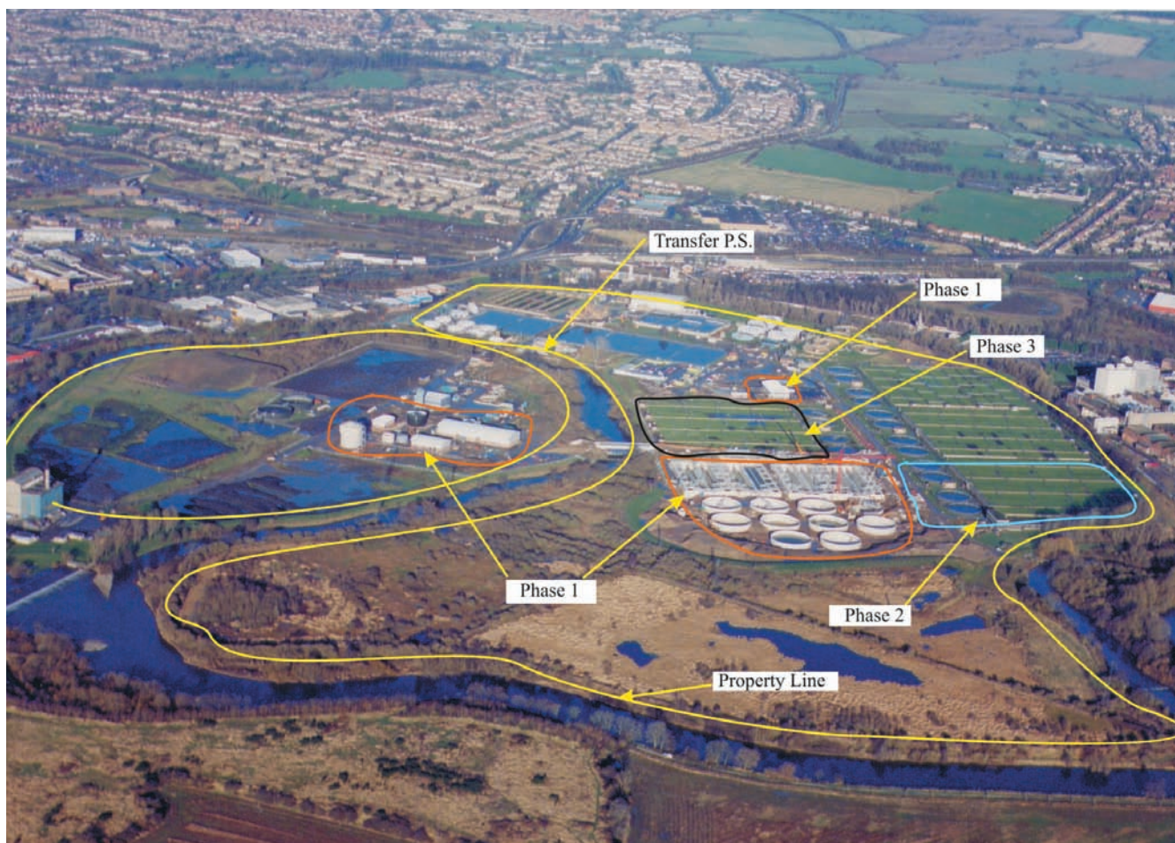
Aerial with site borders etc reimposed (courtesy Severn Trent Water)
