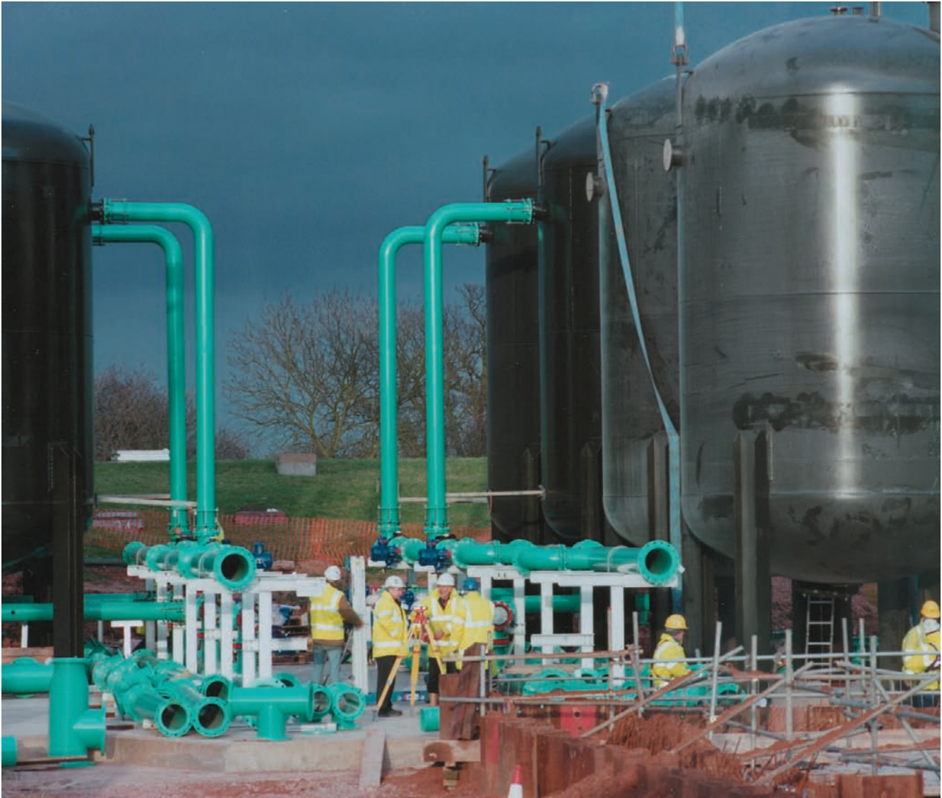
GAC Vessels at Campion Hills WTW (Photo: Stuart Blackwood Photography.Sneinton, Notts; courtesy Severn Trent Water).
