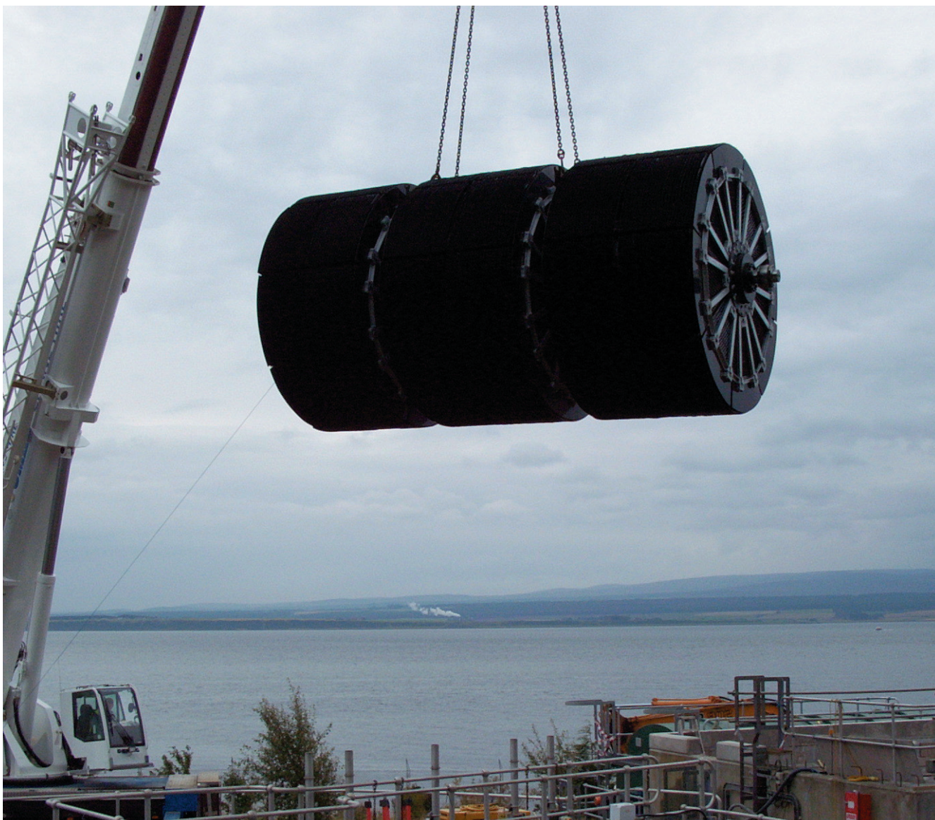
Second rotor installation in modified RC tanks (courtesy Copa Ltd)
