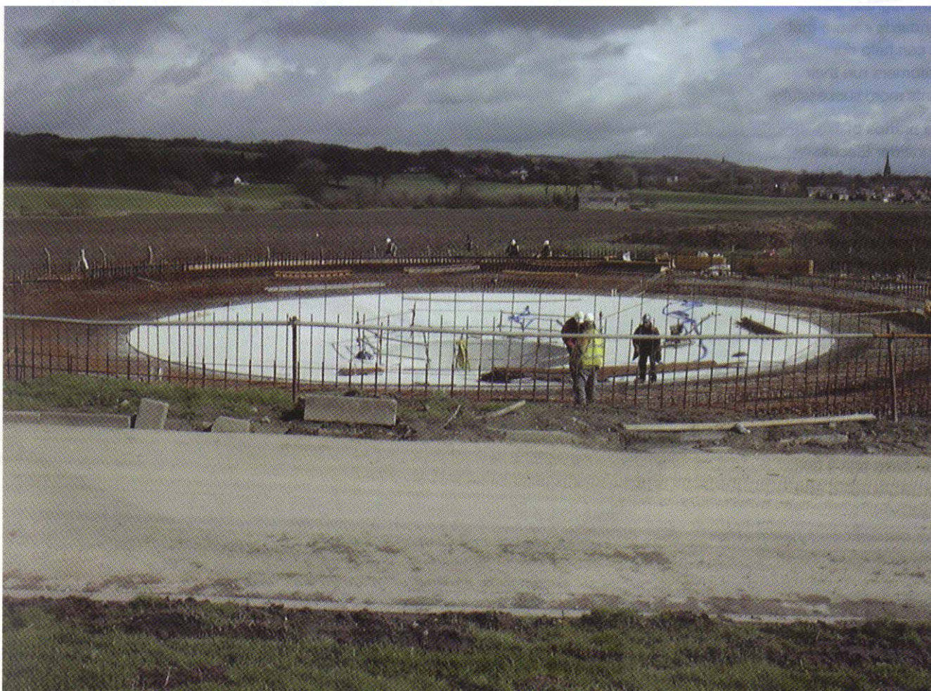
Humus tank under construction (courtesy Montgomery Watson Harza)
