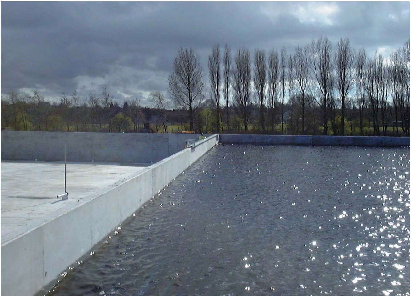
Storm tank with one side under test (courtesy Montgomery Watson Harza)
