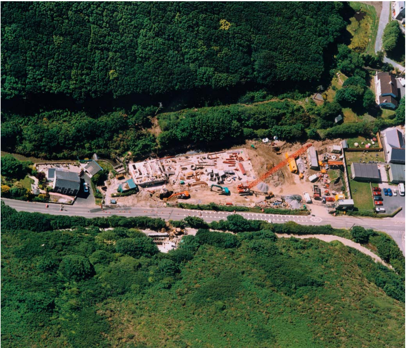
Portreath Pumping Station under construction (photo:: Still Imaging, Chudleigh , Devon; courtesy S.W. Water)
