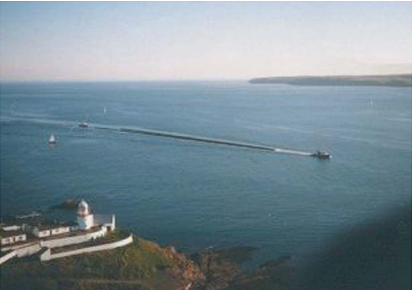
Pipes being towed to Cork Harbour (courtesy E G Pettit & Company).(courtesy E G Pettit & Company)
