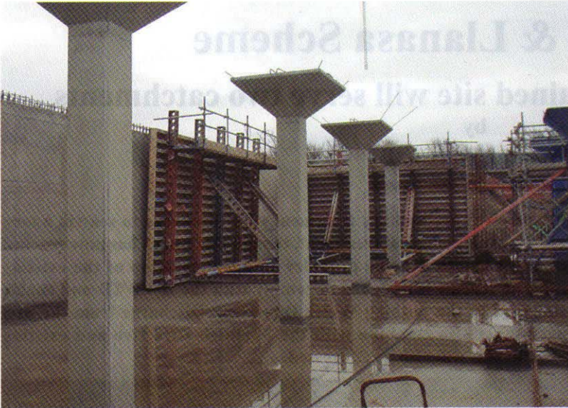
New storm tank under construction at headworks (courtesy E C Harris).
